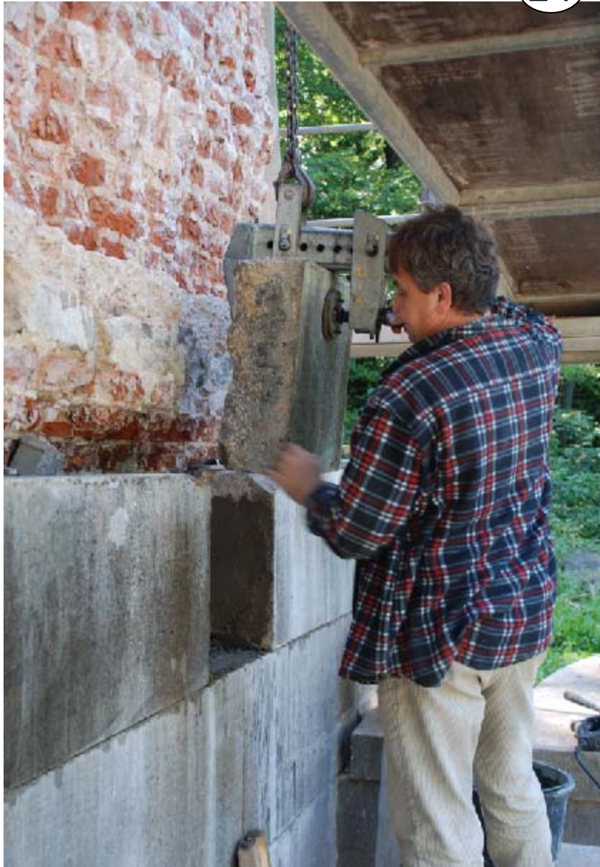
Parts of the walls had to be completely removed and rebuilt
